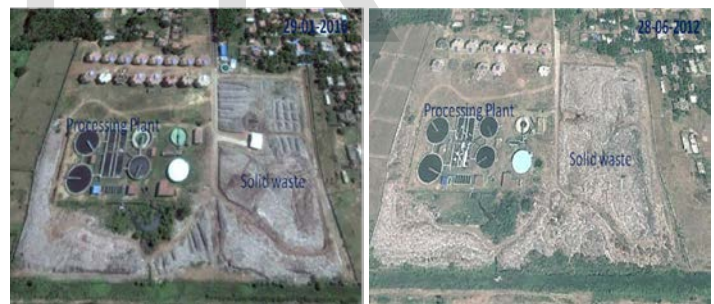
Figure.3. Solid waste dumping Site at Kumbakonam
